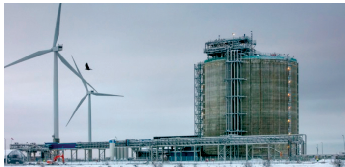
Storage tank at the Skangas terminal in the Port of Tornio
