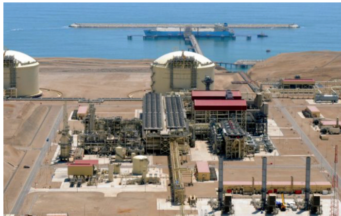
Peru LNG's Pampa Melchorita liquefaction and export plant
