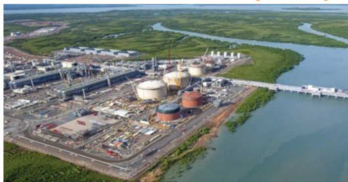
Ichthys project's Bladin Point liquefaction plant near Darwin
