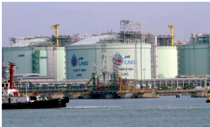
The one existing Thai LNG terminal is at Map Ta Phut
