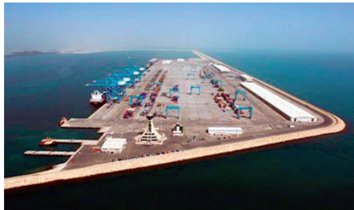
Floating storage to be east of Khalifa Bin Salman port
