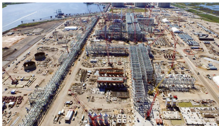
Cameron plant is under construction in Hackberry
