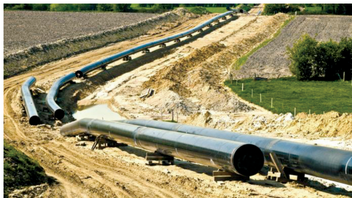
Pipeline expansion work in the southern US state of Georgia
