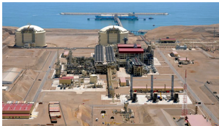
Plant at Pampa Melchorita receives feed-gas from interior
