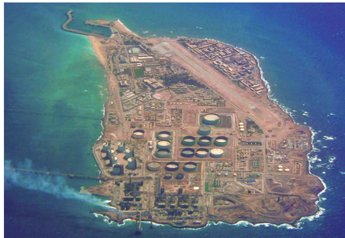
Abu Dhabi has operated LNG export plant since 1977
