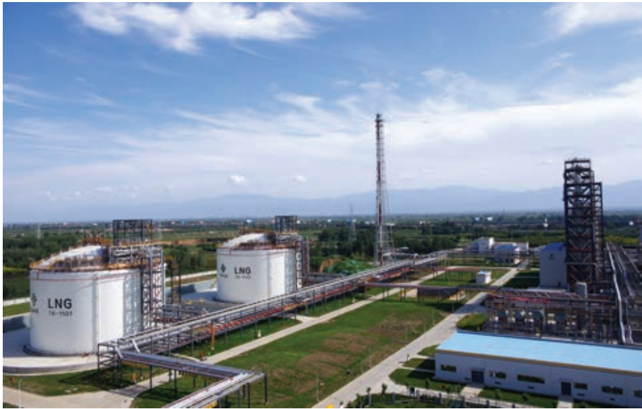
Figure 11: Mid-scale 1350 TPD SMR train
