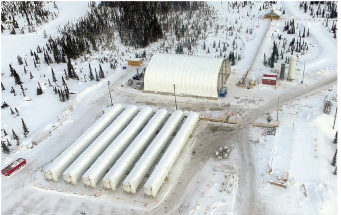
Six horizontal tanks provide LNG storage at a diamond mine in Canada, providing natural gas as the primary fuel
