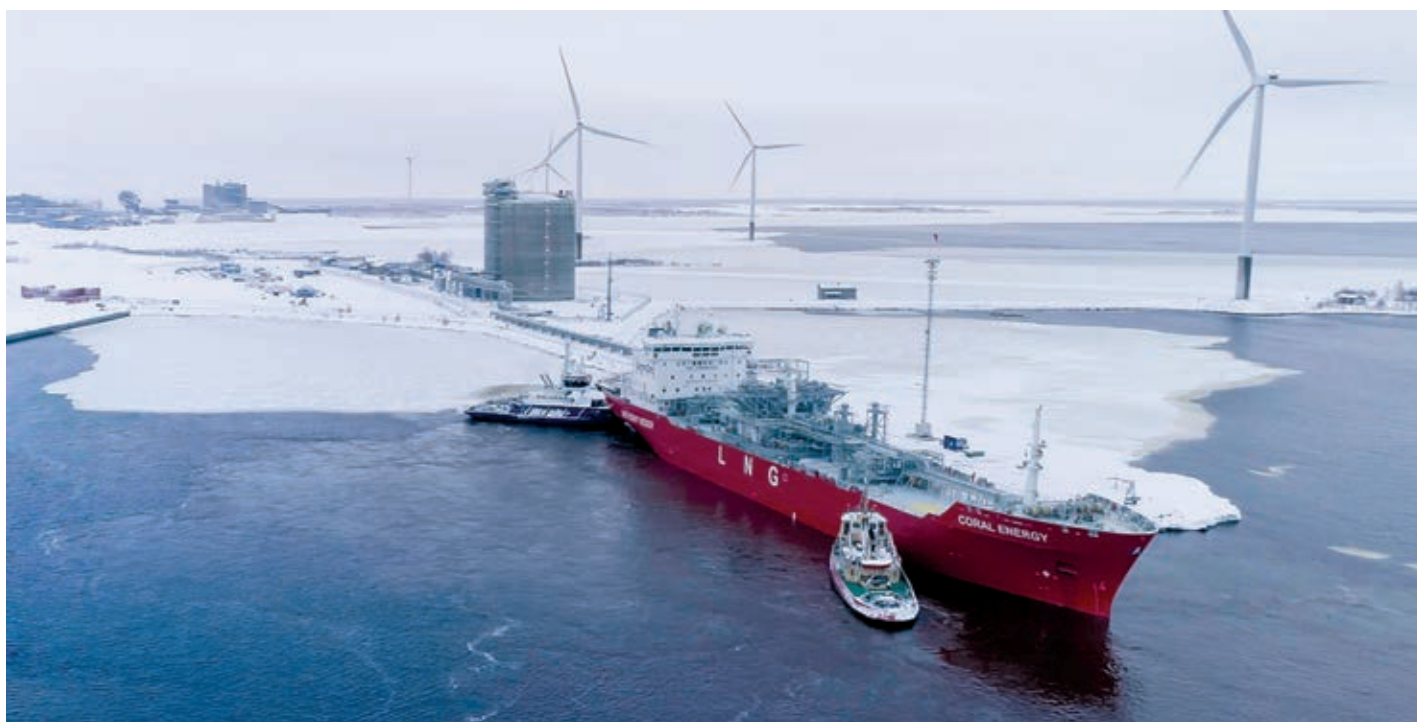
Finland’s Tornio Manga LNG terminal is the nation’s second regas facility to be completed
