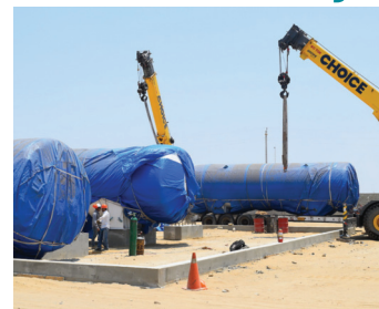
Installation of LNG tanks at the Lanterna site
