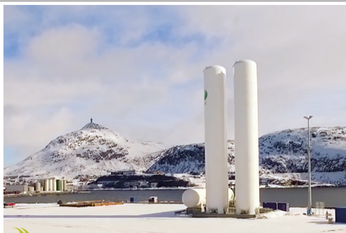
The new Barents NaturGass facility
