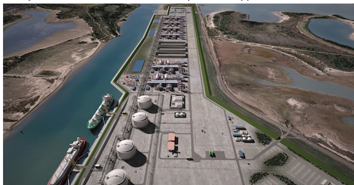
Site of proposed Rio Grande LNG at the Port of Brownsville
