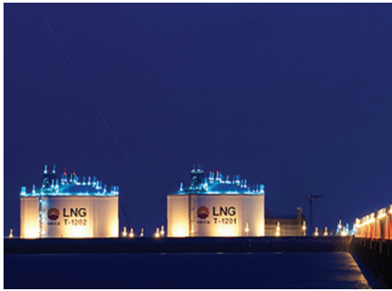
Phase-2 of Rudong terminal is ready
