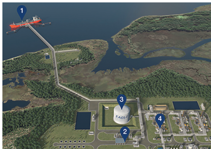
Eagle LNG will point shipments at Caribbean region
