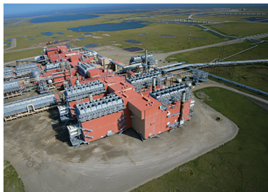
Central gas facility at Prudhoe Bay is part of AGDC plans
