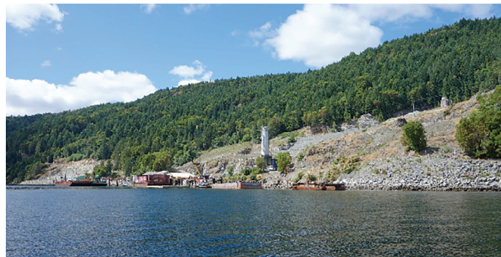
A possible Steelhead LNG plant location in BC
