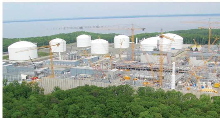
Transformation work well underway at Chesapeake Bay
