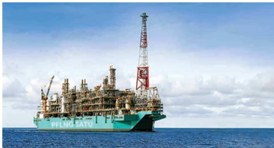
Floating output: 'PFLNG Satu' offshore Sarawak for Malaysia's Petronas
