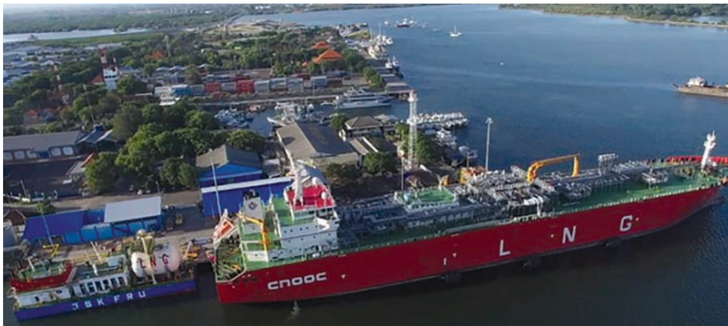
AG&P partner Entec helped set up this LNG facility in Bali, Indonesia
