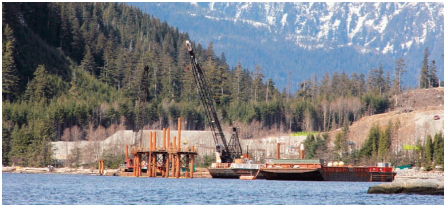
Liquefaction plants are supplied by pipelines hundreds of miles long from inland to the Pacific coast
