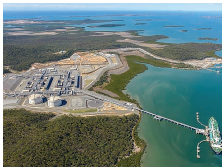
Figure 1: GLNG's two-Train LNG facility located on Curtis Island in Gladstone Harbour, in the eastern state of Queensland (courtesy of GLNG)
