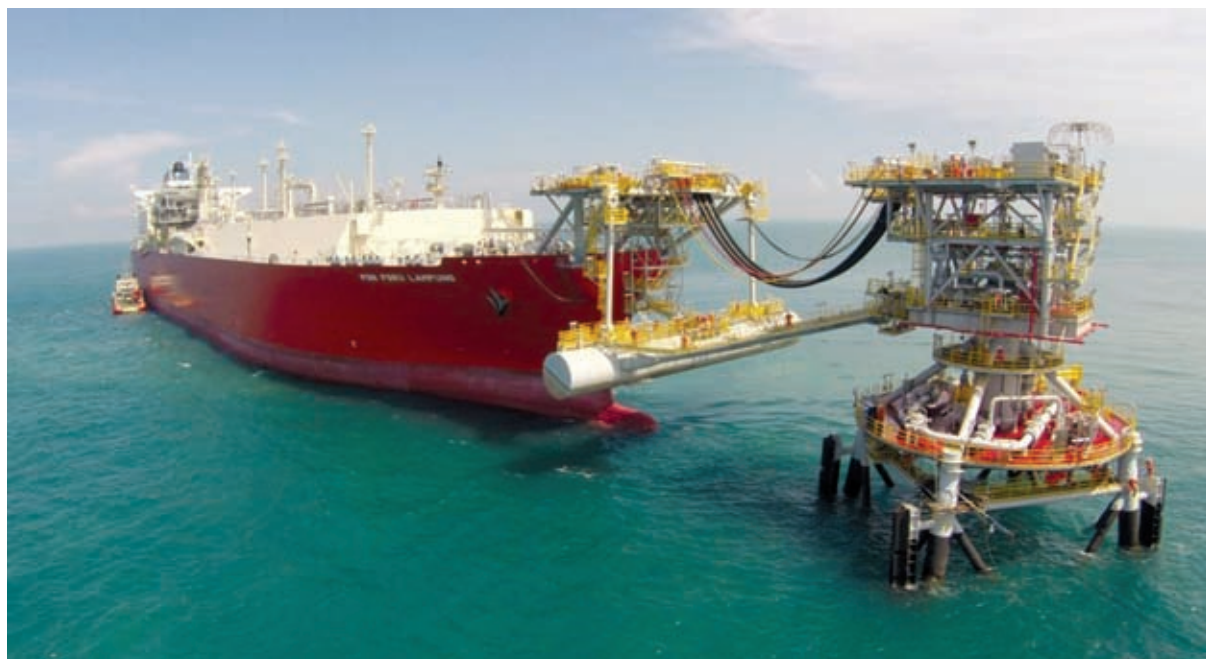
Hoegh LNG's PGN FSRU Lampung was recently hooked up and is now in operation.
