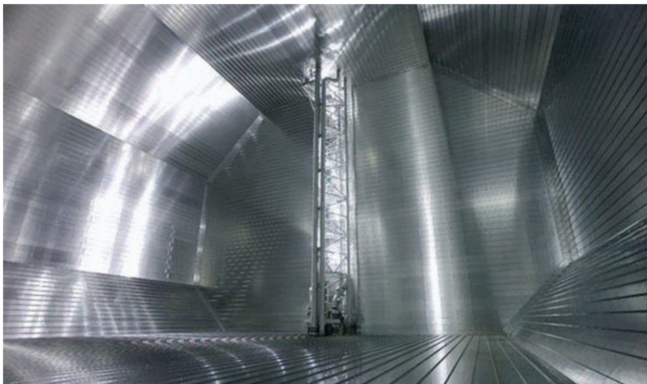
The cavernous area of a membrane tank system is the ideal location for sloshing.
