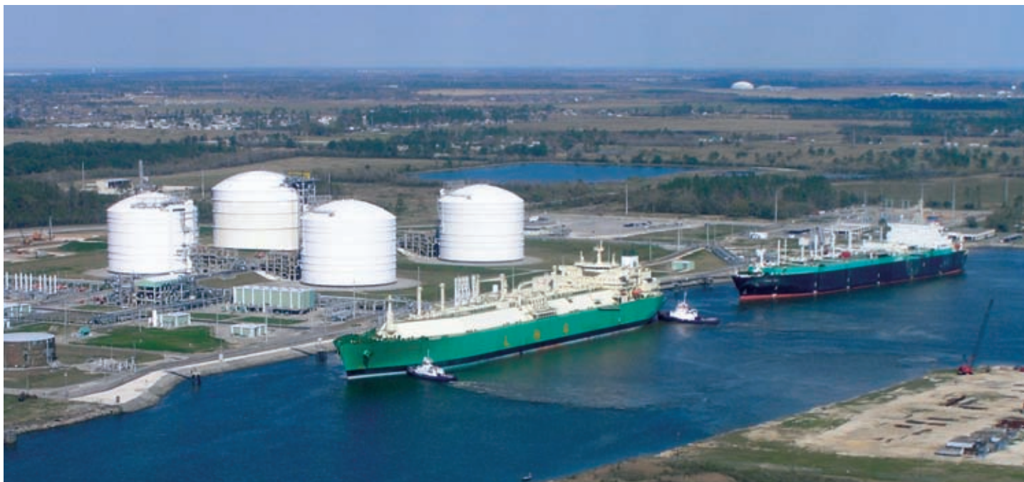
Handling LNGCs in tight situations calls for highly trained personnel in every discipline.
