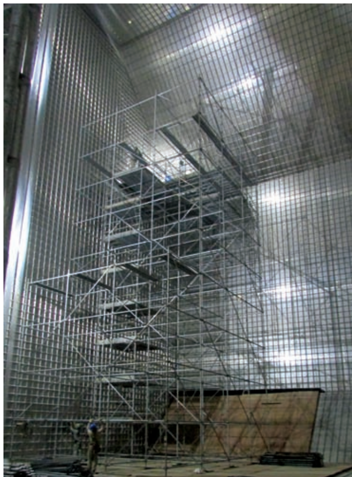
Staging erected inside a gas tank.
