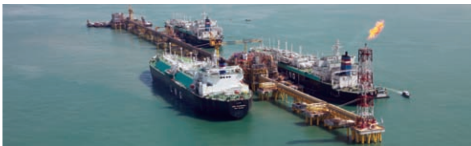
ABS has classed Petronas' Melaka Terminal, which employs an older MISC LNGC as a storage unit connected to a regasification unit on the jetty.
