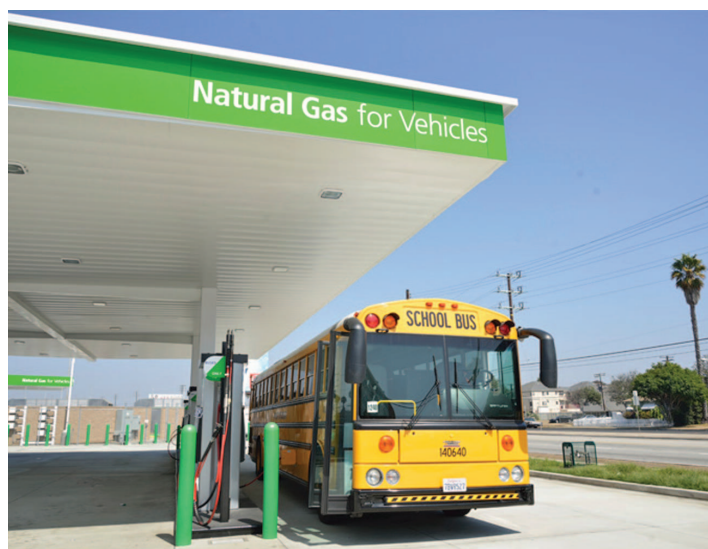
A natural gas filling station Source: Clean Energy Fuels
