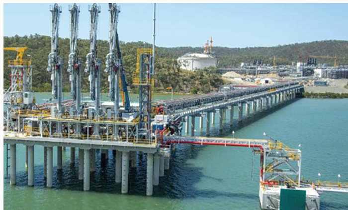
Santos LNG loading jetty at Curtis Island in Queensland
