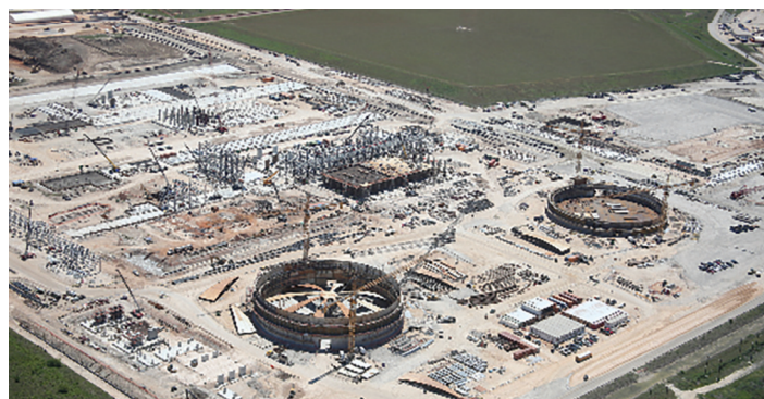
Building underway at the north end of La Quinta Channel
