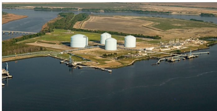
Elba Island LNG terminal to start export plant transition
