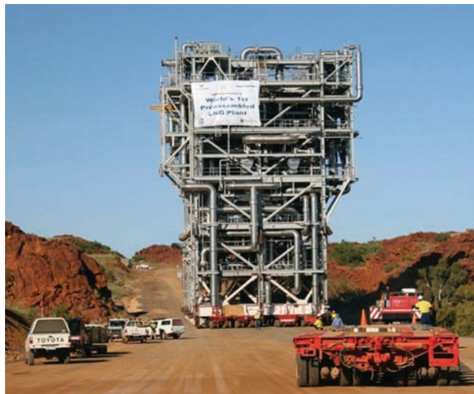
First: NWS Train 5 liquefaction module on the haul road in 2007
