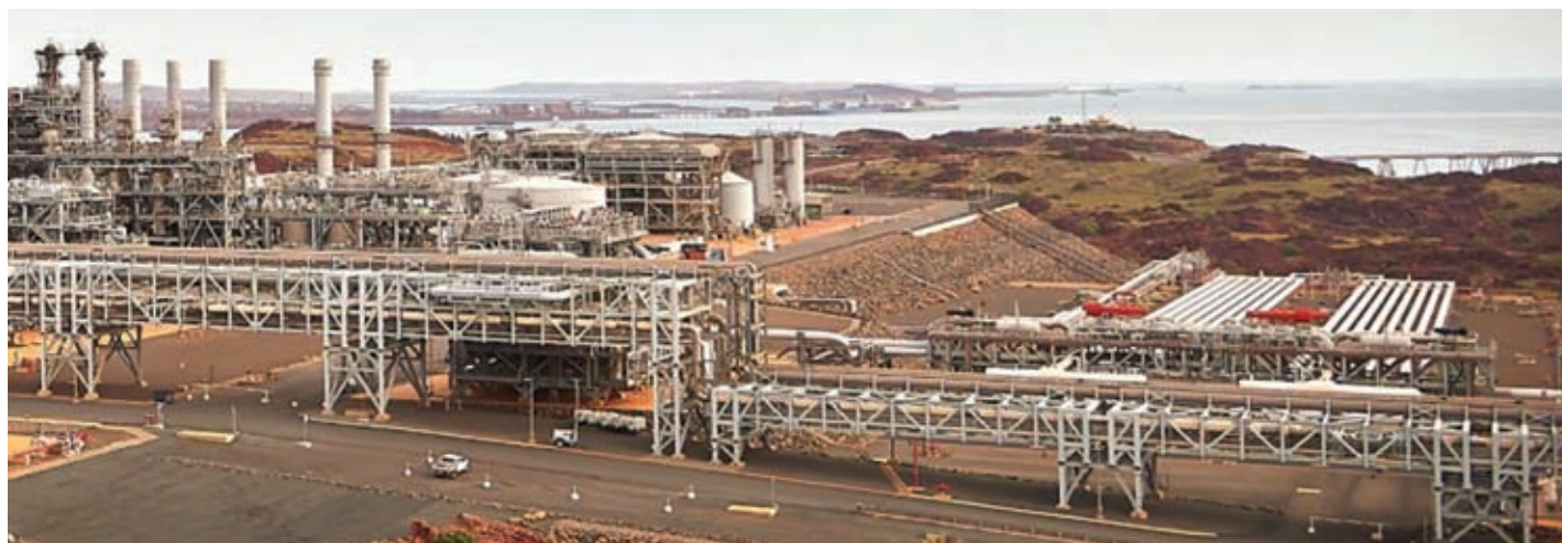
By way of example, Pluto LNG rundown piping was modularised
