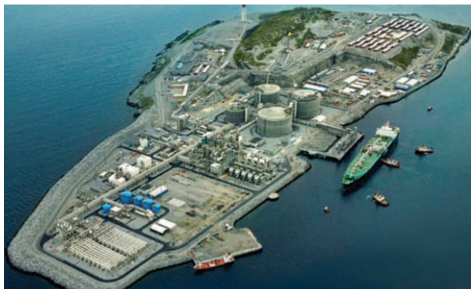
Hammerfest LNG in Northern Norway is connected to the Snøhvit field and is one of six operating plants with gas produced from unitized reservoirs
