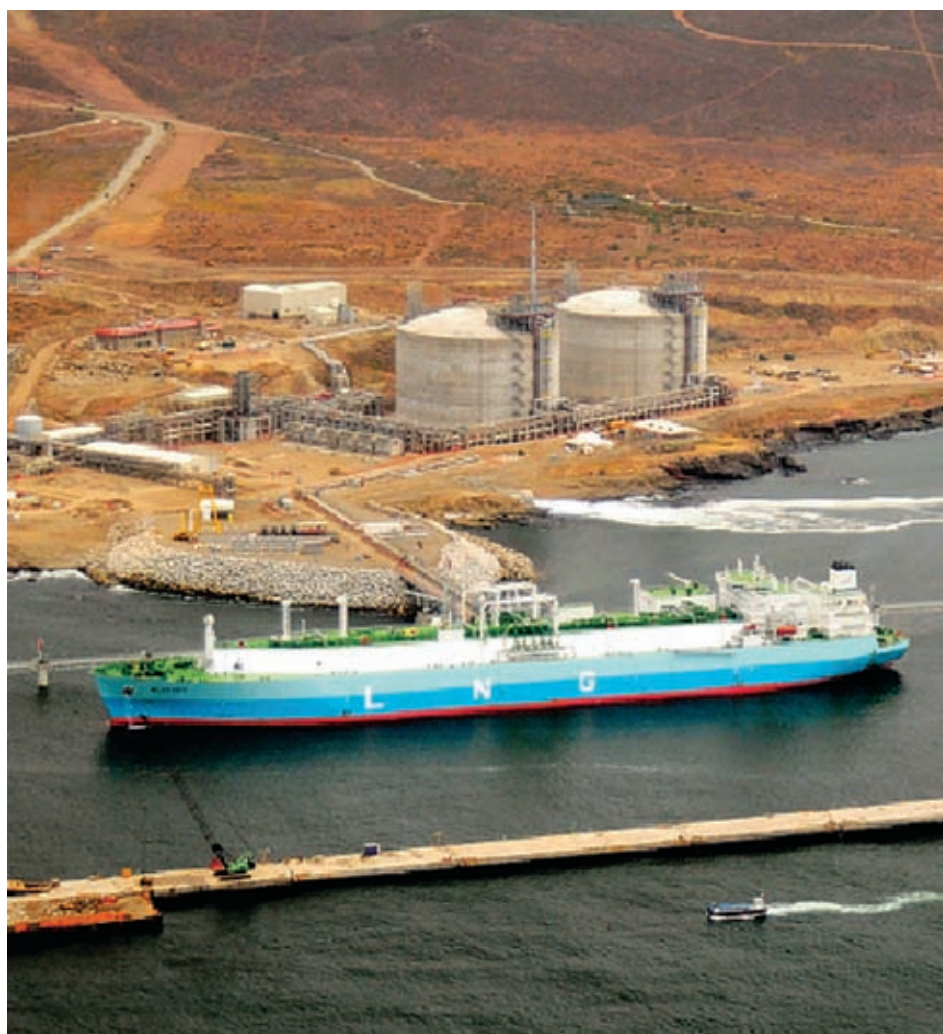
Energia Costa Azul, LNG receiving terminal located in Ensenada, Mexico. It was the first regasification terminal on North America's Pacific Coast
