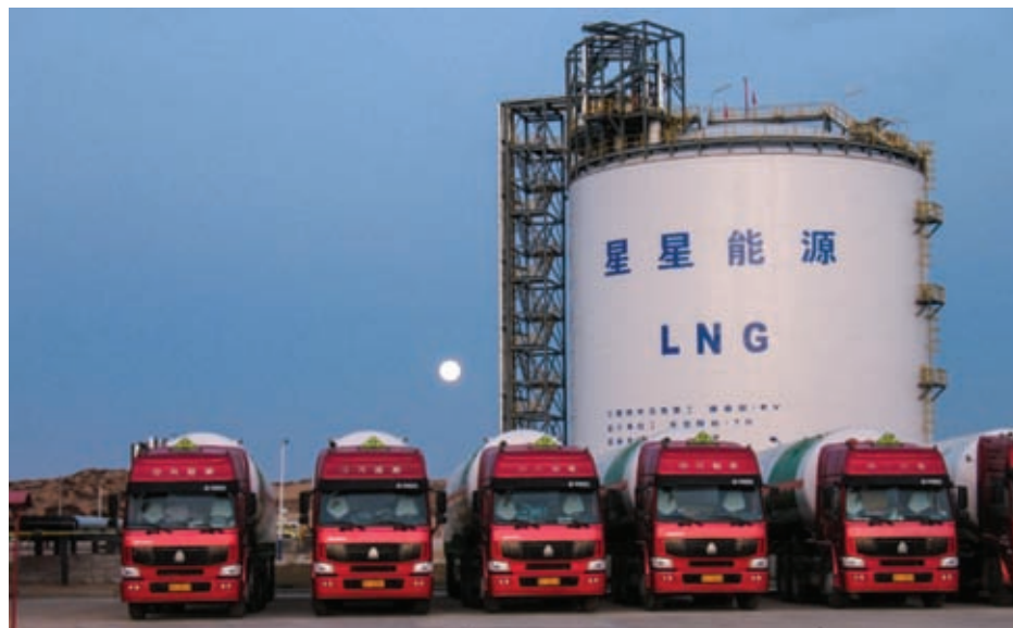
The Erdos facility in Inner Mongolia, China, will produce 200,000 tonnes per year for transportation, industrial and domestic fuel use in the country
