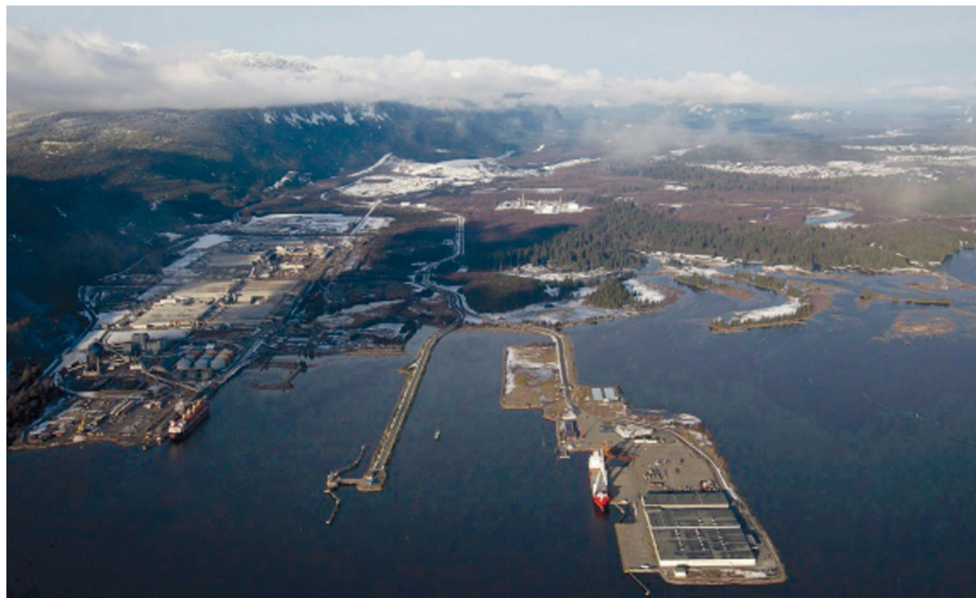
Aerial view of Kitimat, B.C., where Rio Tinto has struck a deal over use of the deep water port with LNG Canada
