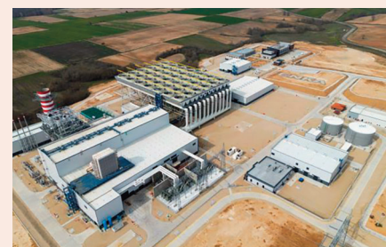
ENKA's Kırklareli power plant, near the Bulgarian border
