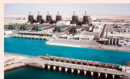
Taweelah B complex in Abu Dhabi
