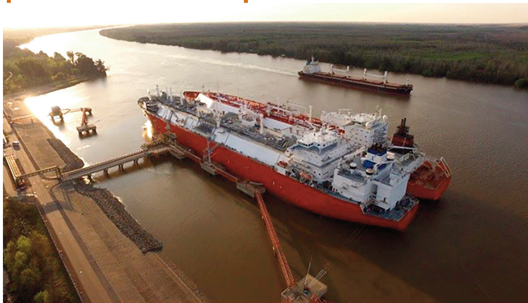
Excelerate-chartered FSRU Escobar connects to the Transportadora Gas del Norte pipeline
