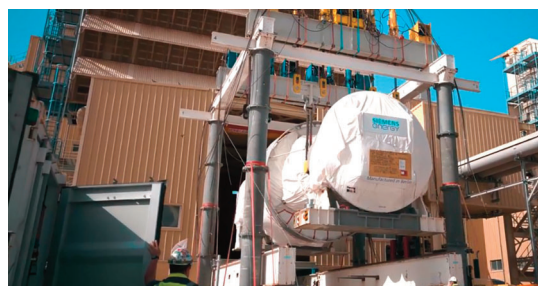
New Siemens turbine arrives at Sarir power plant site
