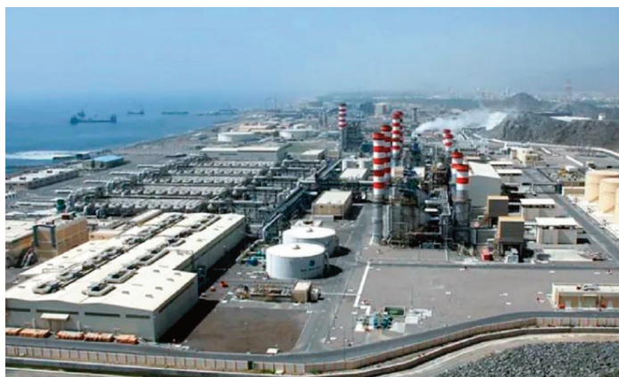
View of Fujarah F1 IWPP in the United Arab Emirates, 40% owned by Sembcorp
