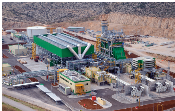
Thisvi CCGT is one of Greece's most modern gas-fuelled
