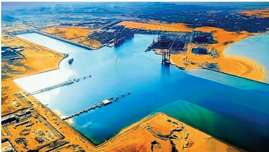
FSRU at Egypt's Ain Sokhna port
