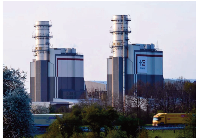
Trianel's H2-ready CCGT project at Hamm
