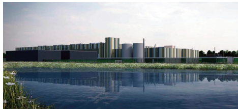
Render of Amazon's data center at Didcot A site
