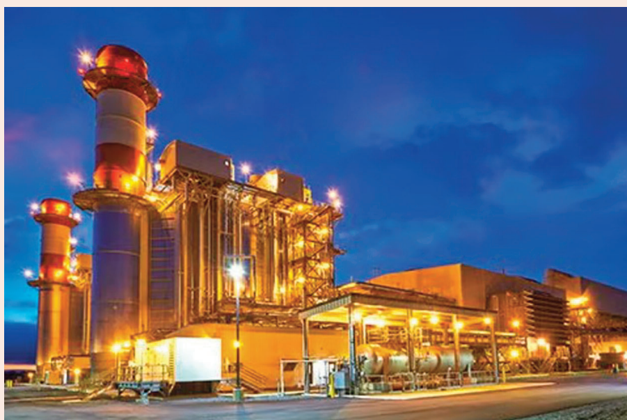
The Patriot CCGT is part of the acquisition
