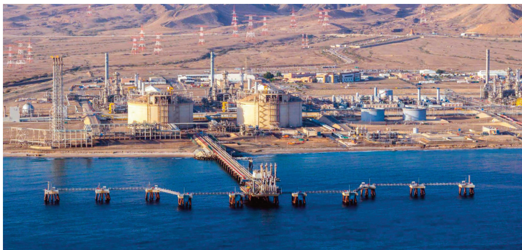
Oman LNG plans to add a third train at its Qalhat complex by 2029
