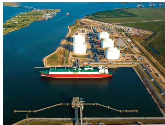
Venture Global's CP2 terminal in Cameron Parish, Louisiana
