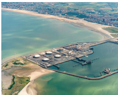
Fluxys' Zeebrugge terminal will have to switch supplies
