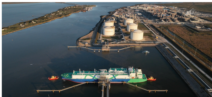
A commissioning cargo is due to be exported later this month
