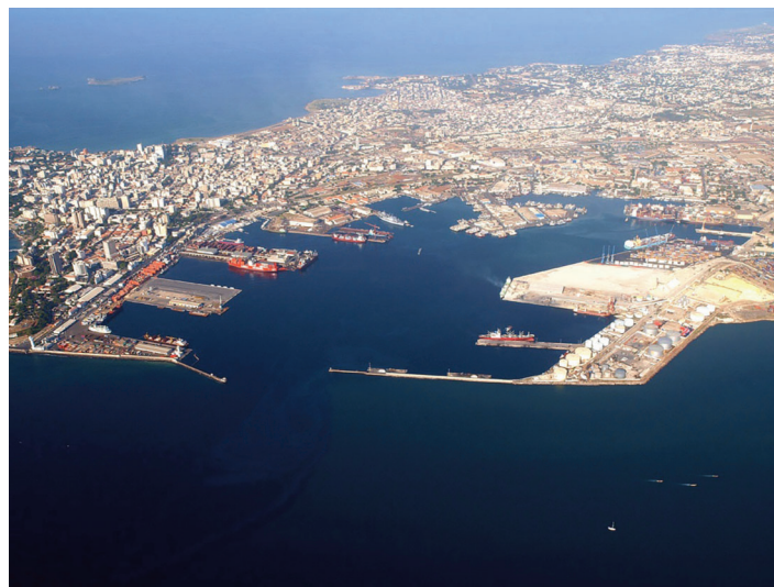
Reganosa is helping to develop Dakar's LNG terminal
