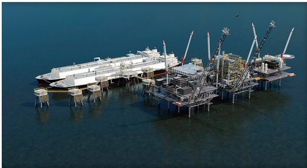
Baker Hughes will supply equipment for ST LNG project
