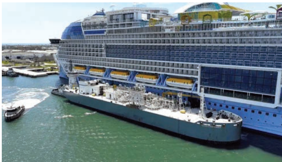
Seaside LNG vessel Clean Everglades during bunkering
