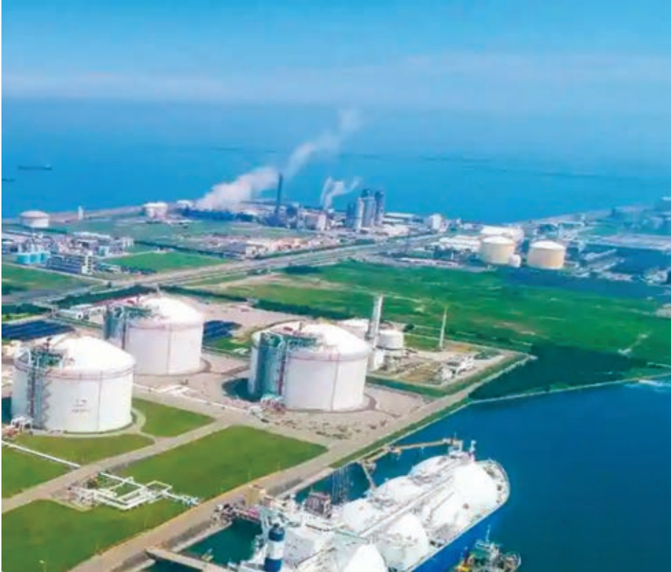
Two LNG storage tanks were added to Petronet’s Dahej terminal, each with 180,000 bcm capacity.
