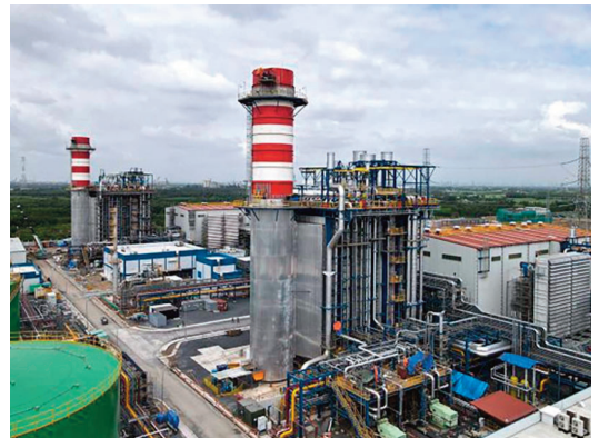
Nhon Trach Units 3&4 are being repowered to LNG
