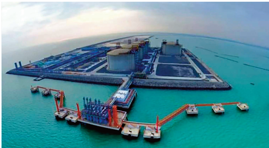
View of Pakistan's largest LNG terminal
